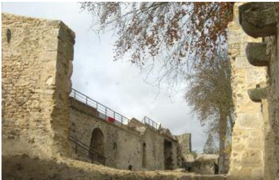
Courtines sud © Yves Morelle
